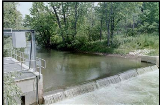
Low head barriers prevent sea lampreys from reaching their spawning grounds, while allowing fish to pass through. They help control sea lampreys without the use of lampricides.
